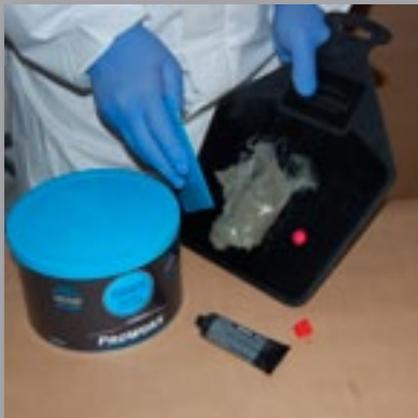
4 Once the area has been prepared, mix your FibreFix filler with hardener at a ratio of 3% at an ambient temp of 20°C.
