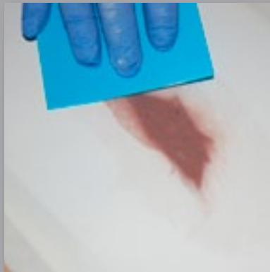
5 Then apply your full coat of filler with the applicator provided making sure that firm and even pressure is being applied.
