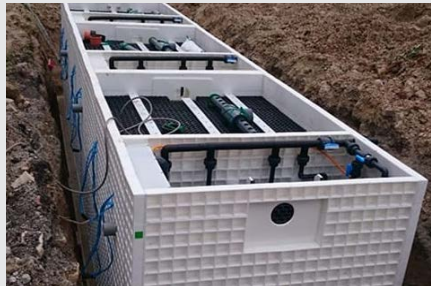
▶ Treatment plant during installation.
