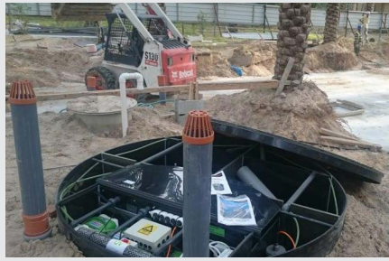
▶ Treatment plant during installation.
